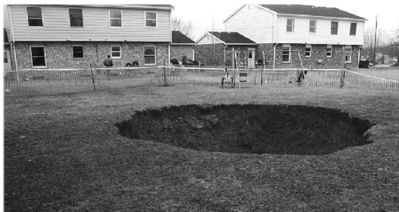
Subsidence pit behind a residence in North Canton, Stark County. This pit was 35 feet in diameter and 25 feet deep. Photo courtesy of Ohio Division of Mines and Reclamation.
